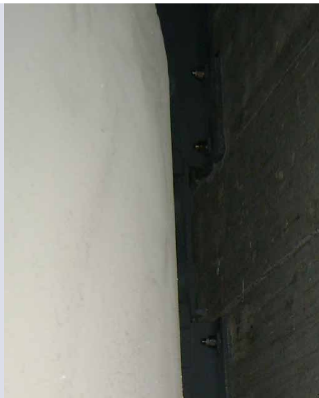
INSTALLATION DE TRANSPORT
